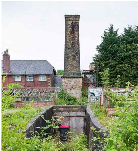
The bothy and chimney
