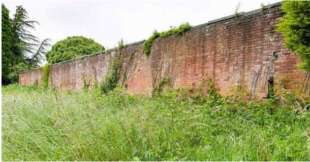
A section of the wall
